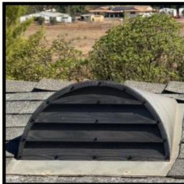
Ember Resistant Mesh Installed Over Existing Roof Vent
