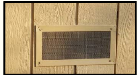
Retrofit Ember Resistant Crawlspace Vent
