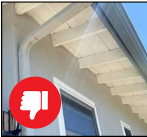
Open Wooden Eaves
